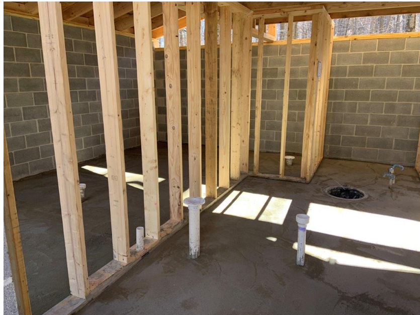
Floor & Studded Walls - March 2023
